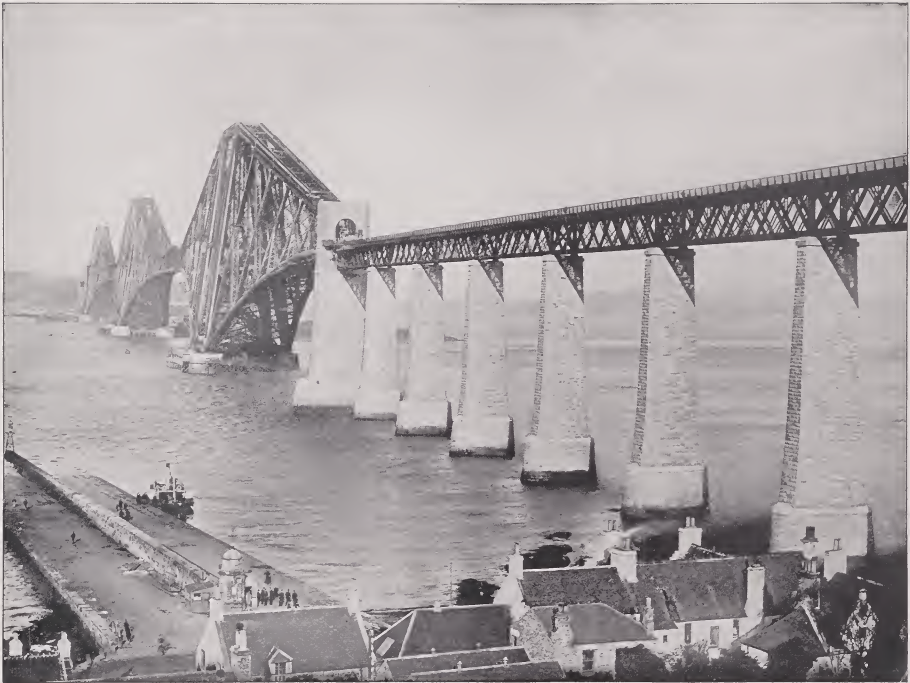
FORTH BRIDGE, SCOTLAND.—This bridge, crossing the Firth of Forth, is pronounced the largest structure in the world, and is the most striking feat yet achieved in bridge-building. It is 8296 feet long, 354 feet high, and cost $12,500,000. It was begun in 1883, and completed in 1890. It is built on the cantilever and central girder system, the principle of which is that of "stable equilibrium," its own weight helping to balance it more firmly in position. Each of the main spans is 1700 feet long, and the deepest foundations are 88 feet. The weight of the metal in the bridge is 50,000 tons.
